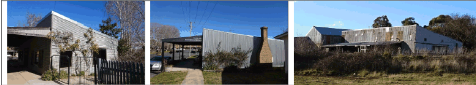
Examples of skillion / lean-to roof forms from within Millthorpe
