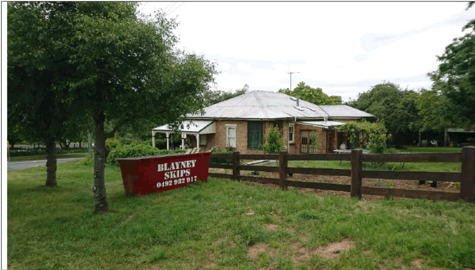
4.3 View of subject site, looking from north-east
